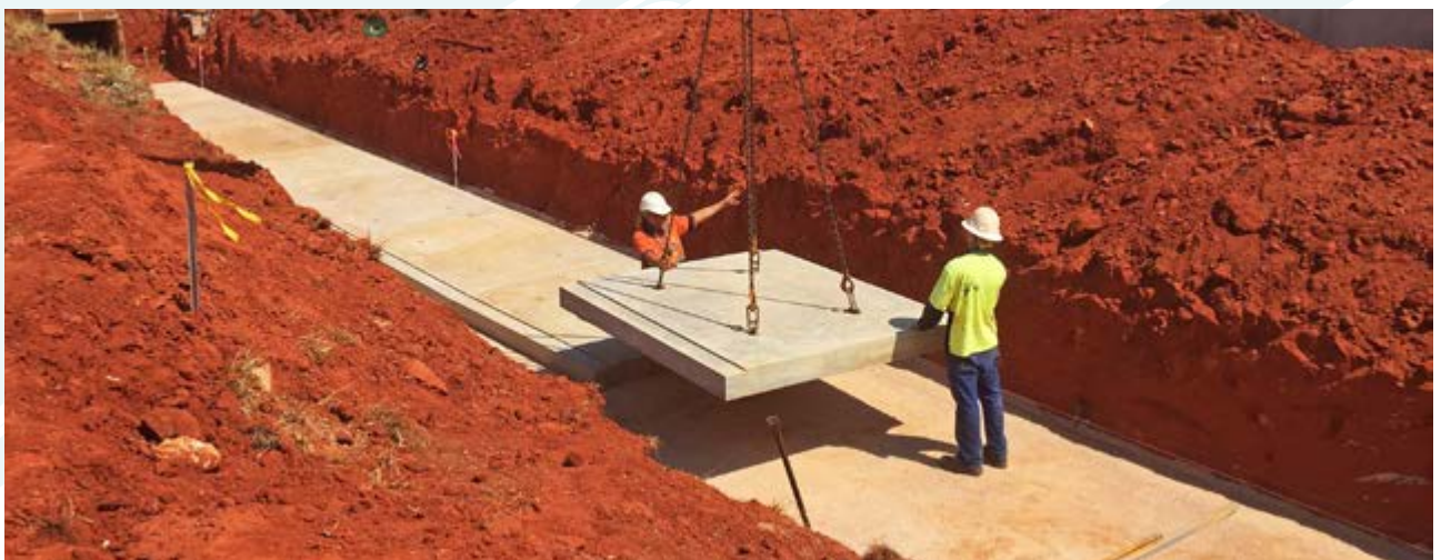
Stormwater drainage near Catalinas at Town Beach is moved underground.
