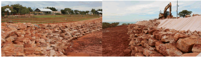
Figure 8.1 Rock Revetments using Kimberly Quartzite north of Town beach (L) and underway at Broome Town Jetty abutment (R).
