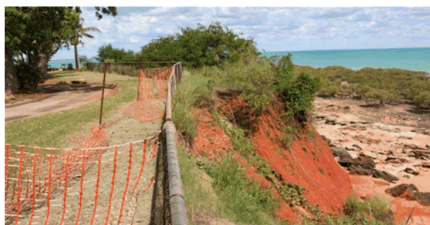
Figure 2.7 Pindan Headland, Fencing and Road within RBCP (Feb 2020), note proximity of fence to crest.
