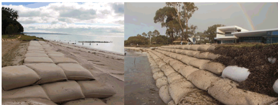
Figure 4.14 Completed GSC Seawall in Busselton.
