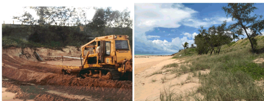
Figure 4.8 Nourishment using beach scraping in front of SLSC looking East following TC Rosita(left) and the same area in Feb 2021 (right) (11).
