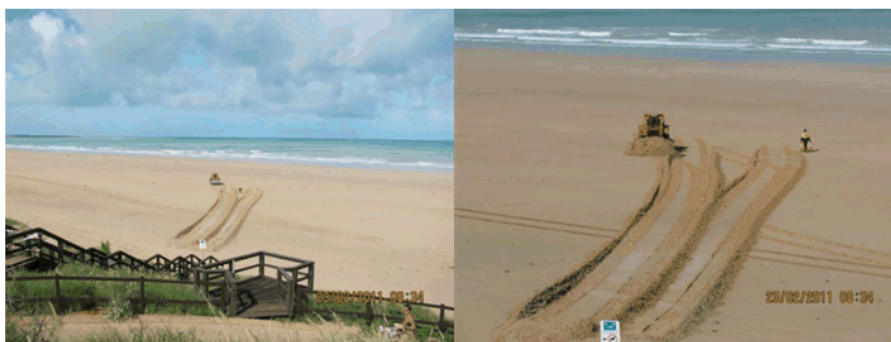
Figure 6.1 Beach Scaping at Cable Beach to Reinststate Foredunes following TC Carlos (Feb 2011)
