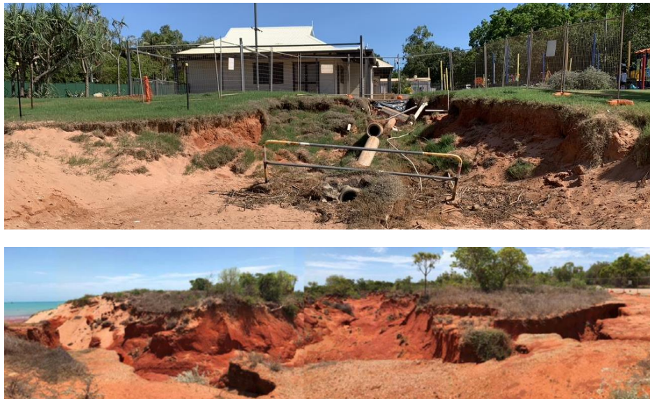
Figure 3.7 – Stormwater Outlet Scour at town Beach in Mar2022 (upper) and Runoff erosion adjacent to Simpsons Beach Carpark, immediately west of Caravan Park, Dec 2018 (lower)
