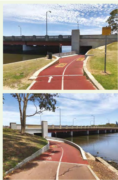
Figure 3.2 Where space constraints result in substandard geometry, advisory measures are recommended to encourage appropriate behaviour by path users.
