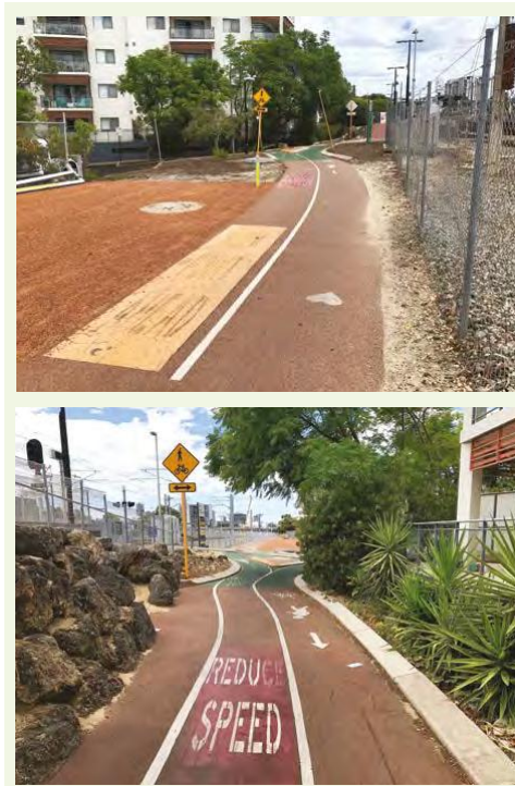
Figure 3.3 Entry point to shared zones, advisory measures are required to highlight the change of use/priority.
