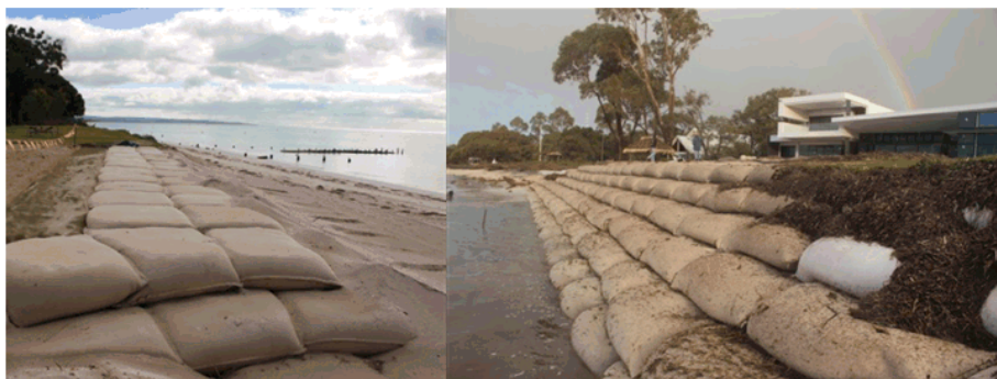
Figure 4.14 Completed GSC Seawall in Busselton.
