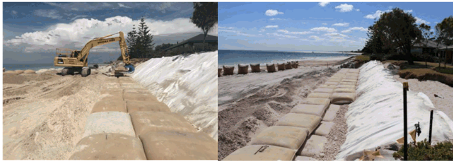
Figure 4.13 GSC Seawall in Busselton under construction (Dec 2020)
