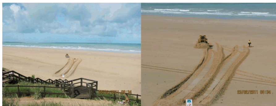
Figure 6.1 Beach Scaping at Cable Beach to Reinstall Foredunes following TC Carlos (Feb 2011)
