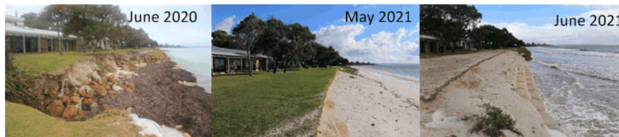
Figure 4.16 GSC Seawall in Busselton. Photos show site prior to construction (left), following construction of Buried GSC seawall and covering with sand (middle), and protection provided by GSC seawall and exposure following storm (right).
