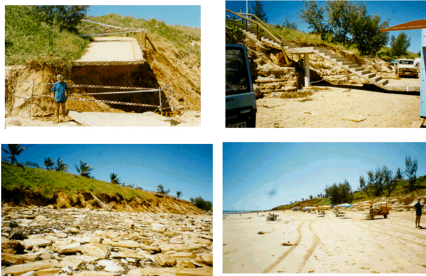
Figure 3.6 Cable Beach Following TC Rosita (April 2000) (images show damage to access ramp and undermining of stairs (upper) and scoured beach (lower) (11)
